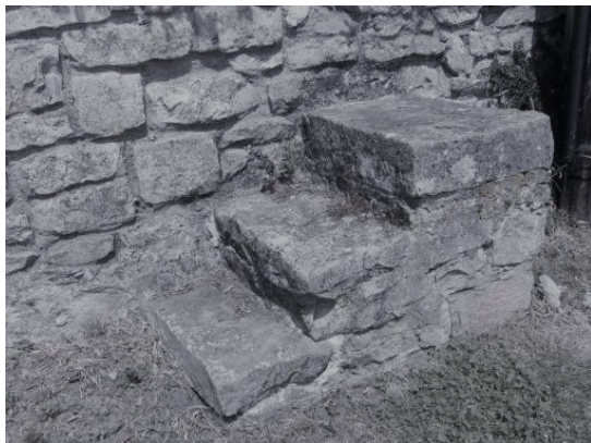
Left: Mounting block outside Village House
