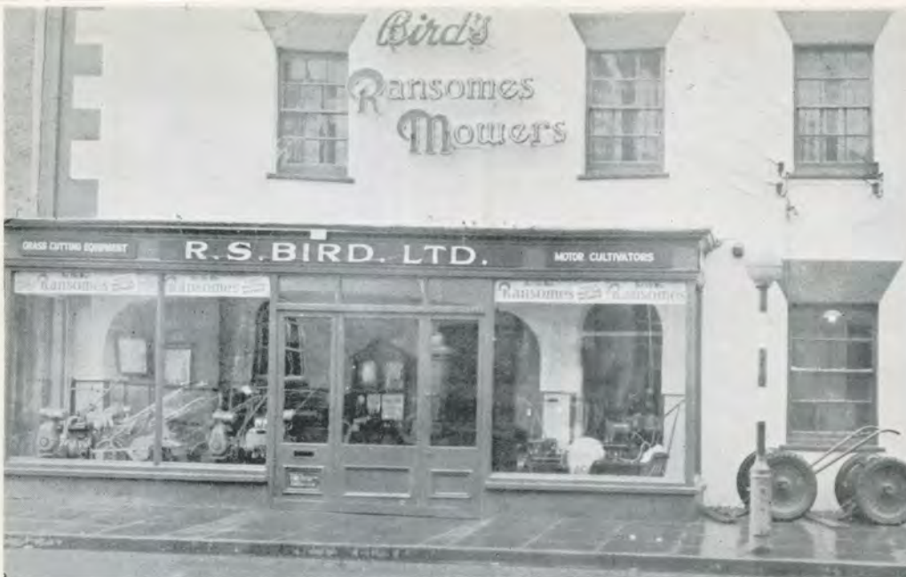
The old showroom known to every traveller to the West, now in course of reconstruction
