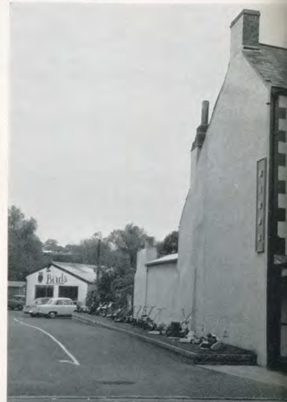
The new entrance to the works in High Street, Cowbridge.
