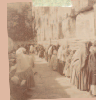
Mur yr Wylofaen Wailing Wall
